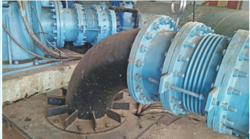
Discharge Head of SubVT Pump
